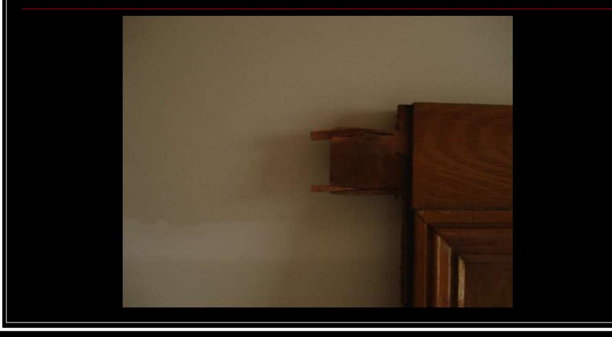
The tongue was split top & bottom and wedges driven in to tighten – and no glue was used – and it held since 1860!
